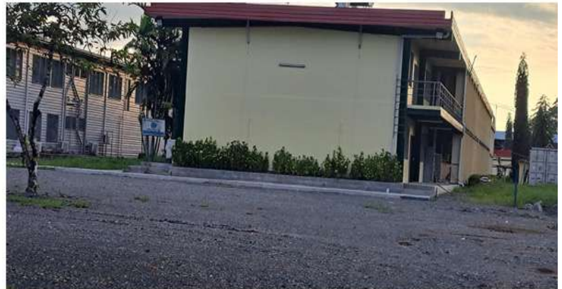
Car Park upgrade and west wing of the Radiological Laboratory
