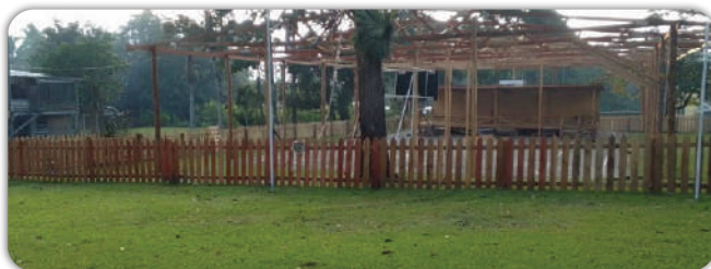
Figure 1a. Temporary hall constructed
